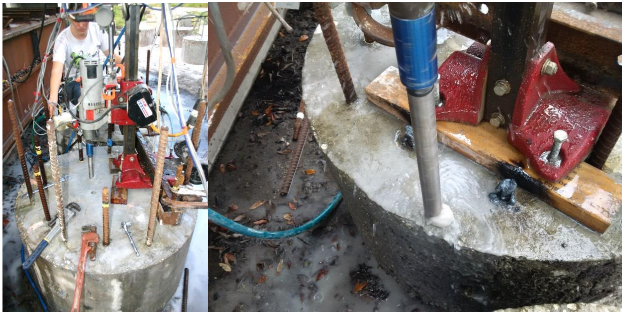
Figure 3.71-Coring inside (left); outside cage (rt), both show coring after extension was added.
