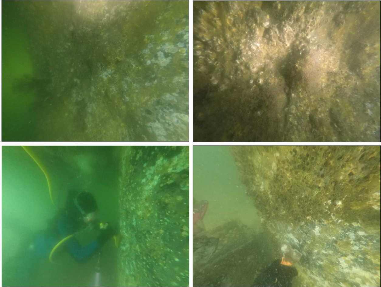
Figure 3.90 As-found and cleaned surface of shafts from Pier 95.
