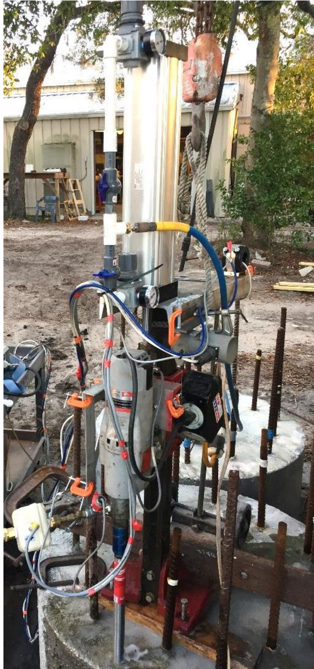
Figure 3.70- In position, prior to coring with 14in starter core barrel.
